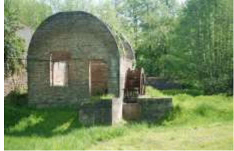
Water powered gunpowder mill
